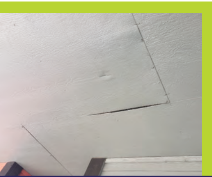
Look for gaps and buckling as shown in this image.
